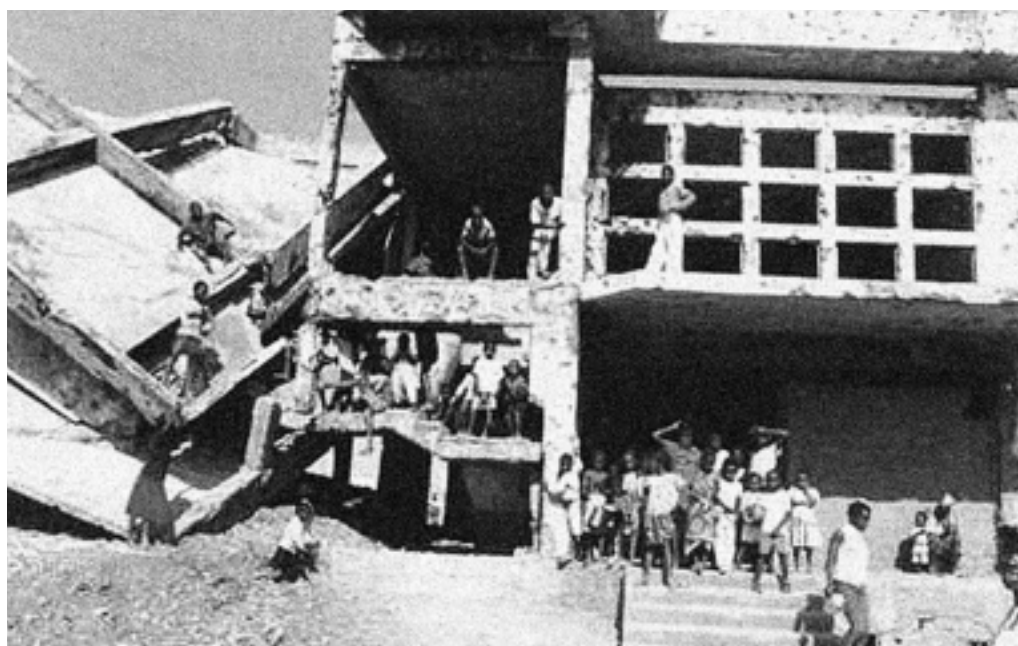
Against all the odds and lack of funds—a functioning Angolan school
